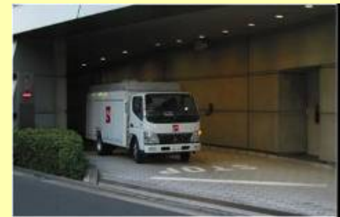
Entry/exit control at public parking areas
