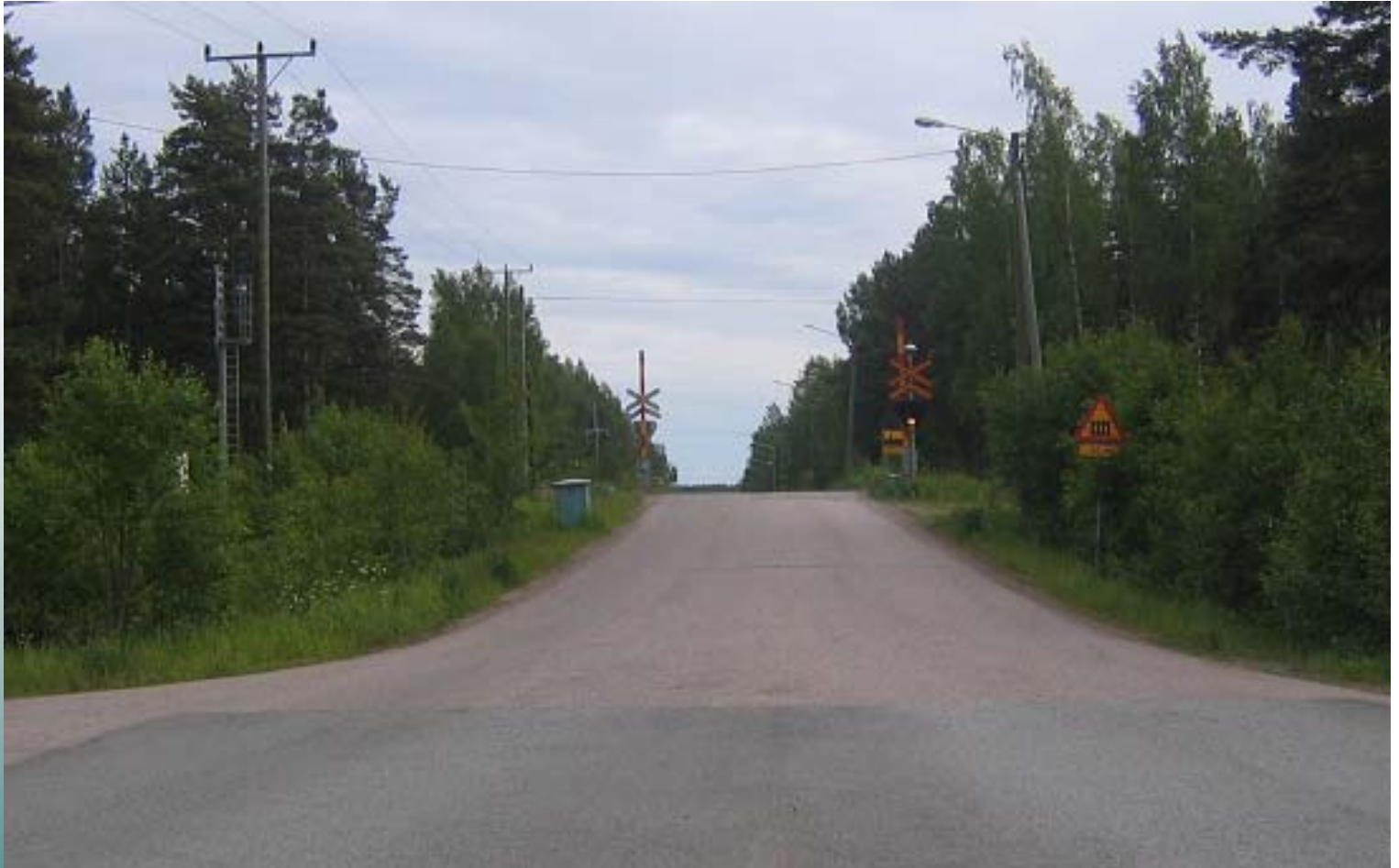
Lappohjan satama level crossing, Hanko
