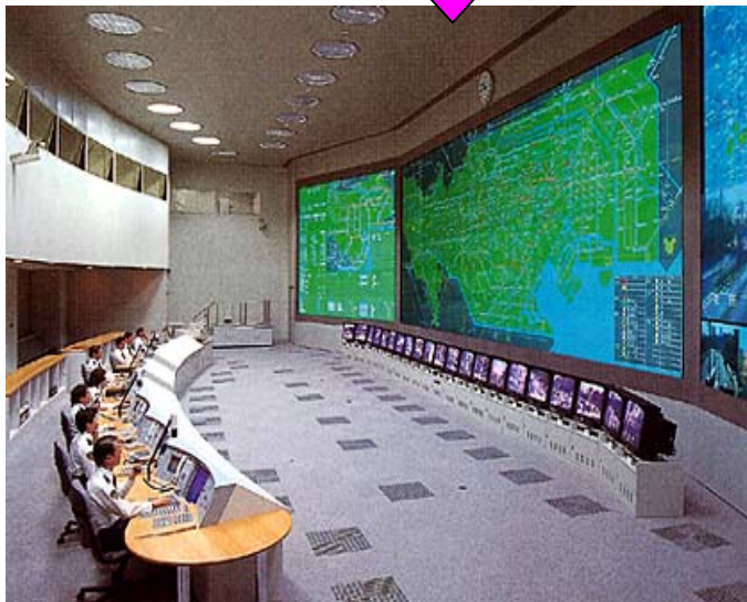
Traffic Control Center
